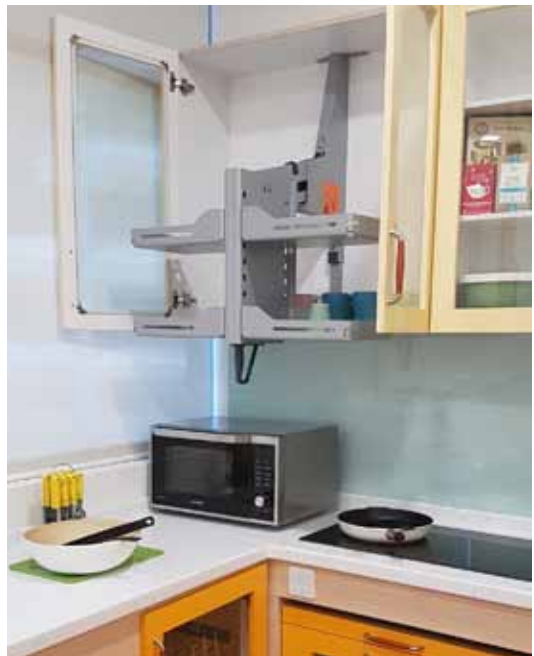
Photo 12: Height-adjustable kitchen cabinet
