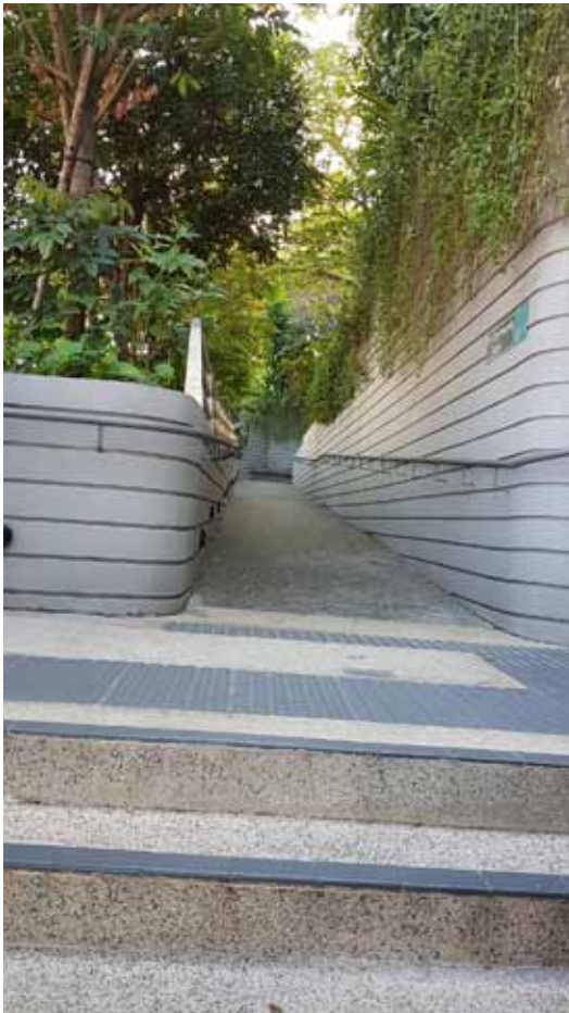
Photo 39: Steps at the base of the ramp at the Rooftop Community Farm
