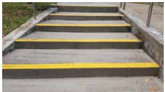
Photo 32: Steps marked with yellow paint/ strips (I'DGO 2014)
