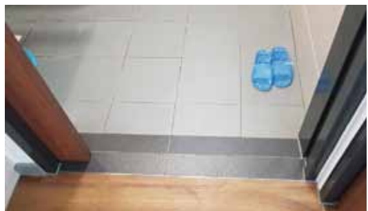
Photo 13: Ramp at the bathroom-toilet entrance
