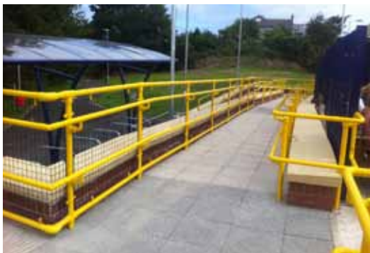
Photo 30: Handrails along the ramp (source: https://www.roofedge.co.uk/news/story/access-for-all-with-key-access-fittings )
