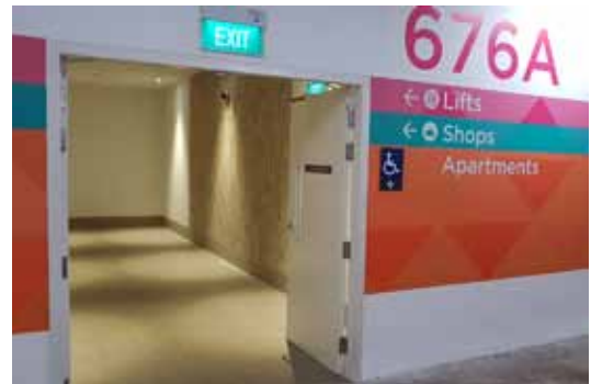
Photo 24: Doors to lift lobby and signage at the carpark of residential block 676A
